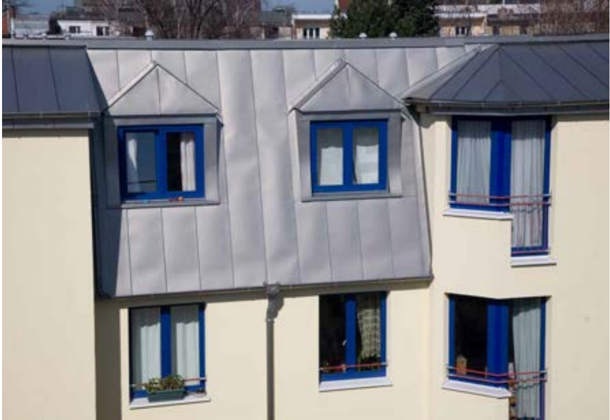
Visible oil canning on a sunny day
