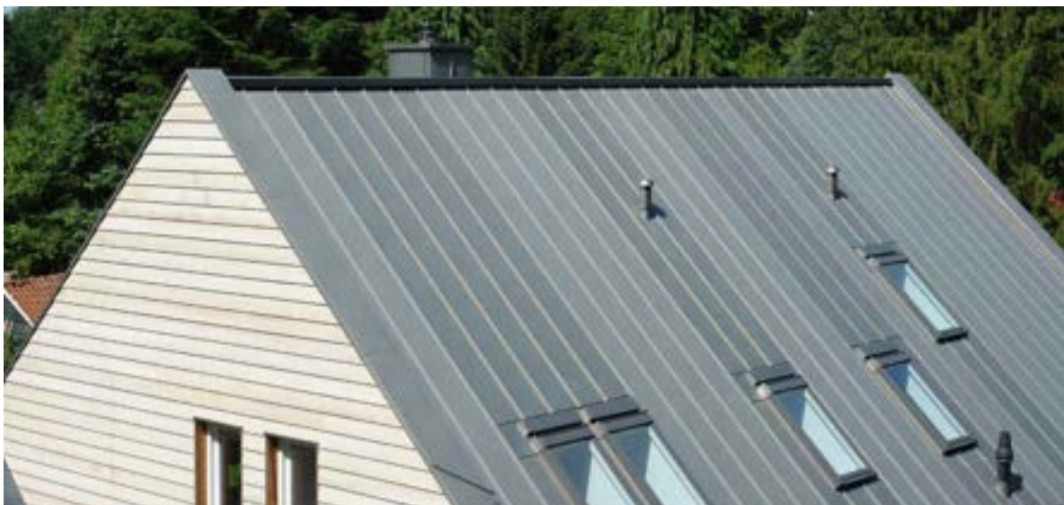
Colour differences on a pitched roof
