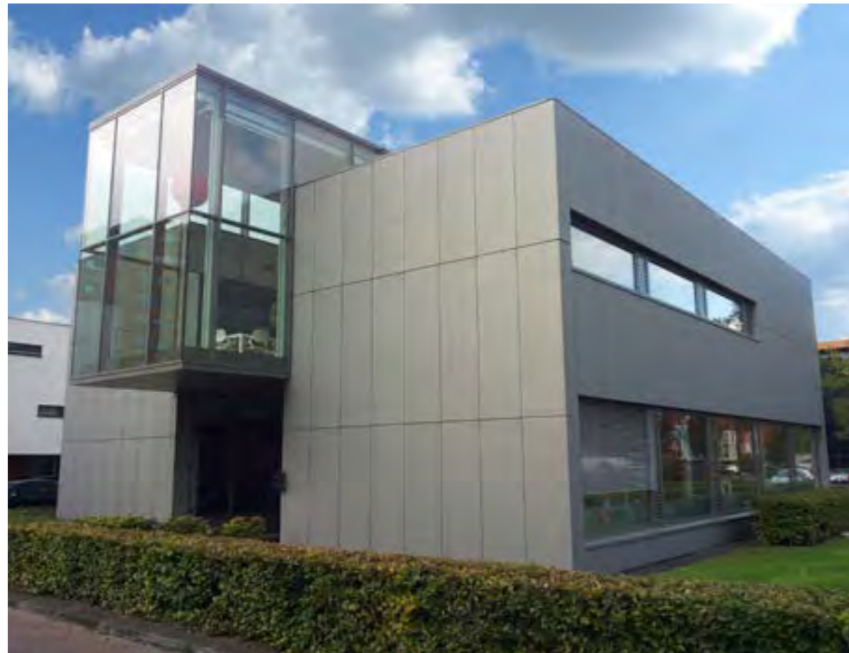
Damp proof façade built up with NedZink reveal panel system.
